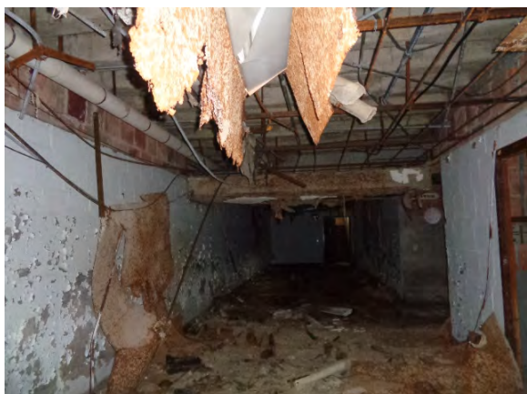
Damaged ACM Plaster and TSI Debris in Basement
