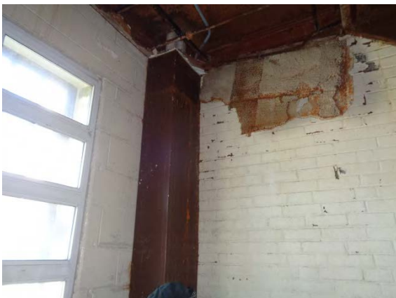
Vertical Pipe Chase with ACM Pipe Insulation in Stairwells
