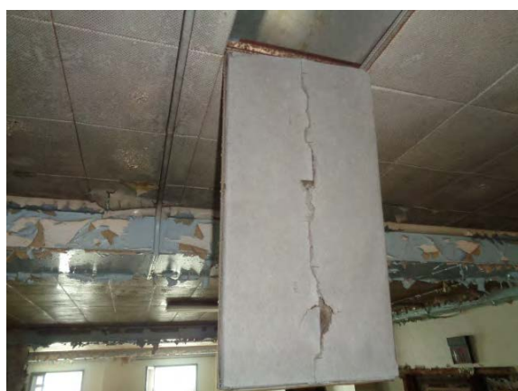
ACM Gray Paper Wrap on Metal 1' x 2' Ceiling Tile Insulation
