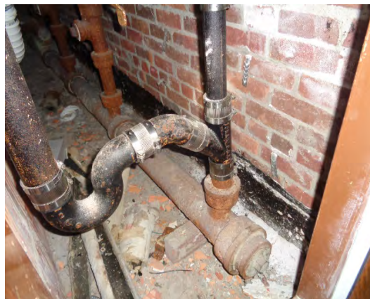
ACM Black Damproofing/Tar/Paper in Bathroom Wall Pipe Chase
