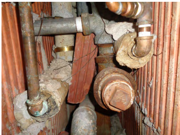
ACM Pipe Insulation in Wall Pipe Chase
