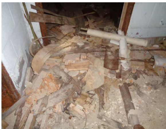
Damaged ACM TSI Debris
