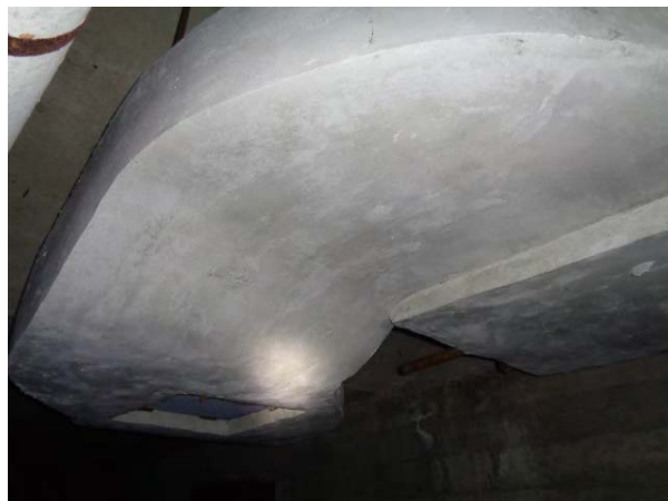
ACM HVAC Duct Insulation
