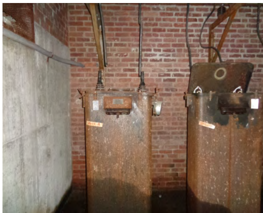
Universal Waste Transformer Oil Reservoirs in Basement
