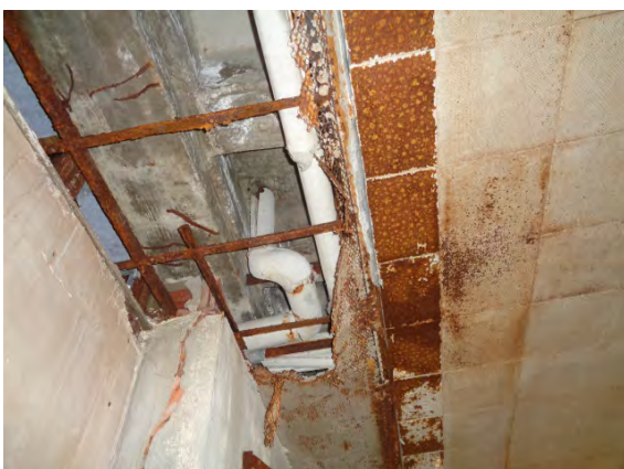
ACM Pipe Insulation and Mudded Pipe Fitting Insulation above Ceiling
