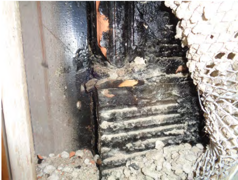
ACM Black Tar/Damproofing on Terracotta Block
