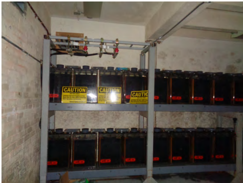
Batteries with Fluid (Corrosives) in Basement
