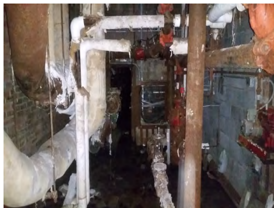
ACM Pipe and Mudded Pipe Fitting Insulations in Basement
