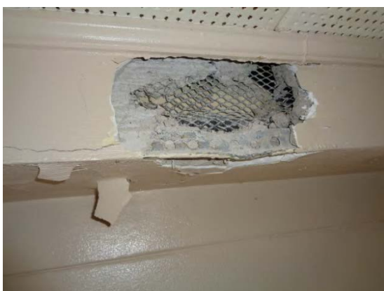
ACM Pipe Insulation in Concealed Horizontal Ceiling Pipe Chase
