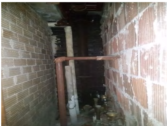
ACM Pipe and Pipe Fitting Insulations in Wall
