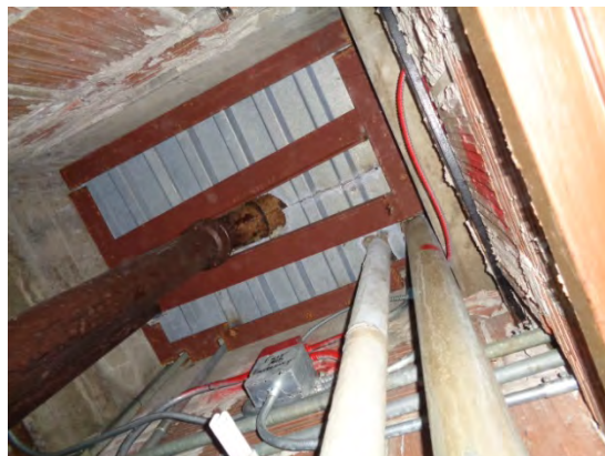
Wall Chase with ACM Pipe Insulation
