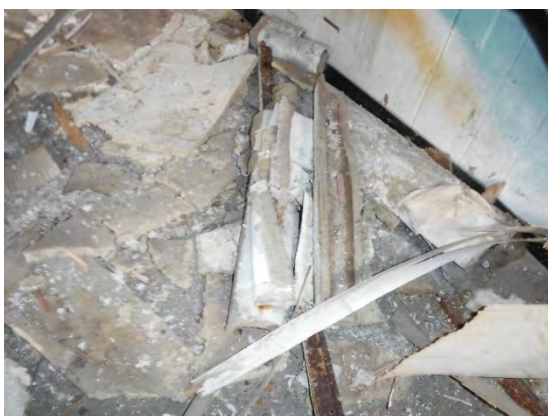
ACM Thermal System Insulation Debris
