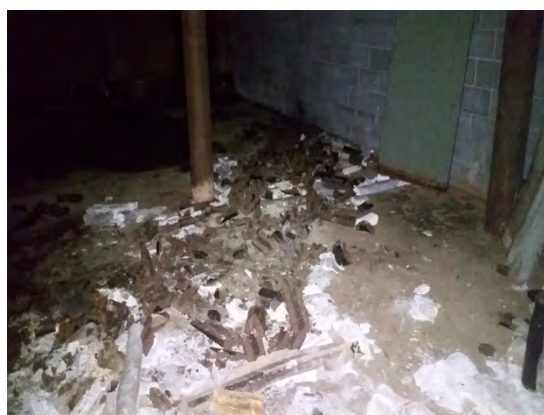
ACM Thermal System Insulation Debris on Basement Floor
