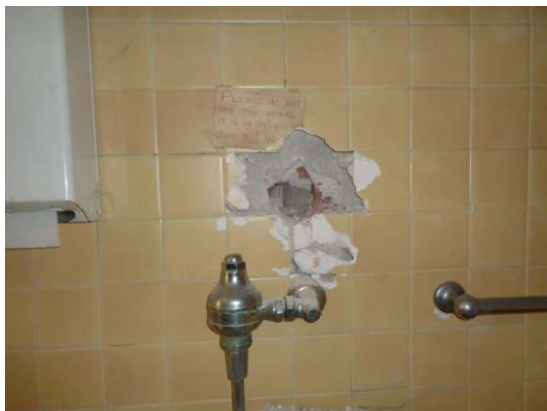
Concealed ACM Pipe Insulation in Bathroom Wall
