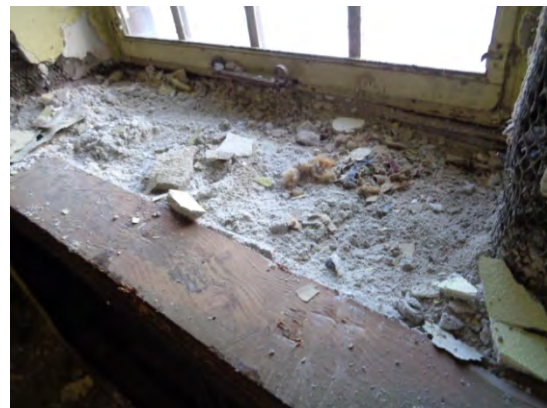
ACM Packing Insulation around Radiator
