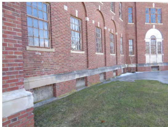
Exterior Window Systems with ACM Window Glazing Compounds
