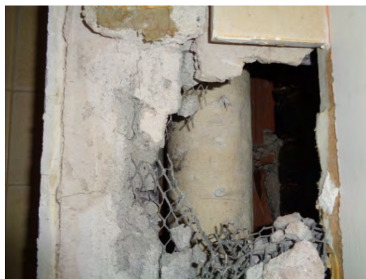
Concealed ACM Pipe Insulation in Vertical Pipe Chase
