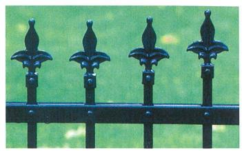
Material: Brick and monumental iron fence, provide ball top on pickets for safety or use monumental iron fence with flush/flat top.
