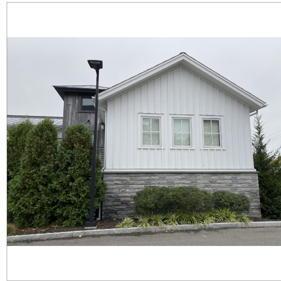
VERTICAL "BOARD & BATTEN" SIDING
