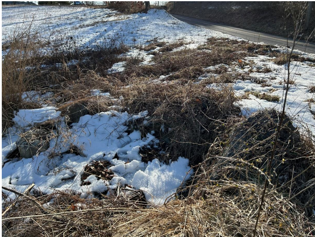
Photo 1 – Town Drainage Pipe Outlet (from Castle Hill Road)
